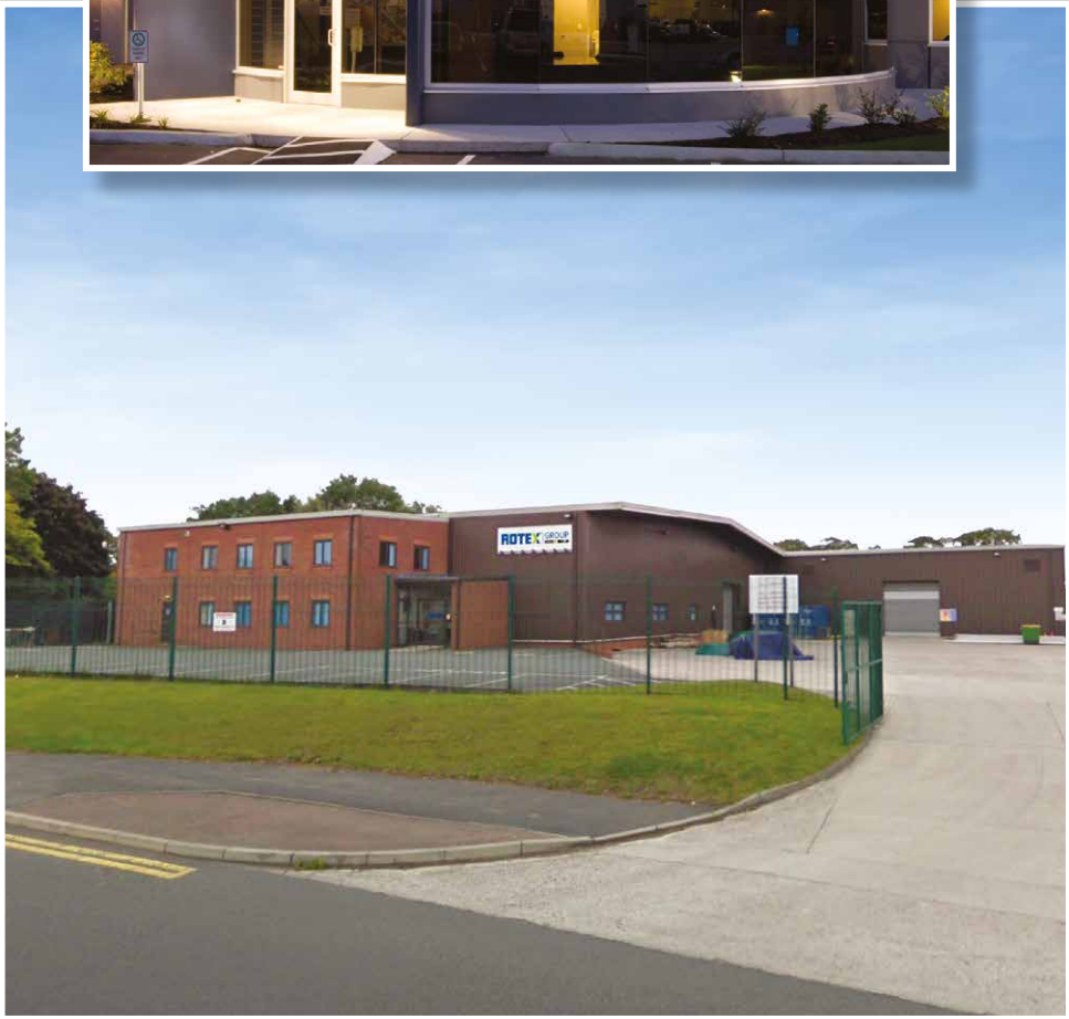
Rotex Europe facility in Runcorn, England, UK
